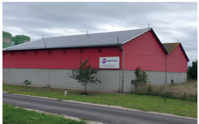
Solar panels at UM Argos Feed in Hungary
